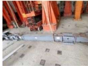
(b) Demount second-story frame
