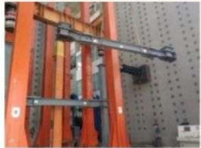
(a) Second-story frame lifting
