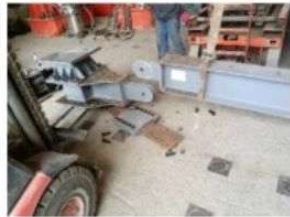
(e) Disassemble the steel beam
