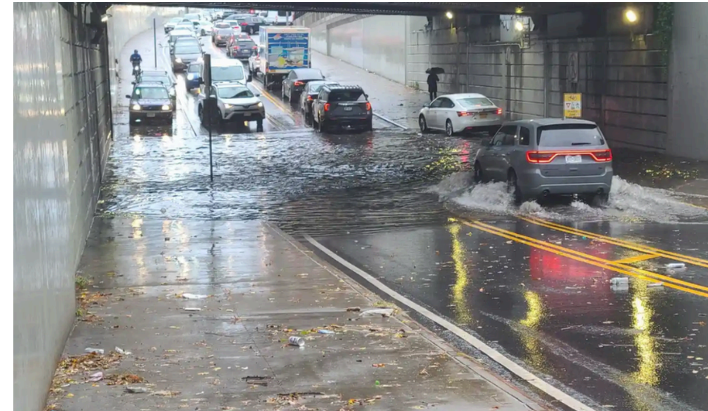
The Cooper Avenue underpass in Glendale flooded on Oct. 30
