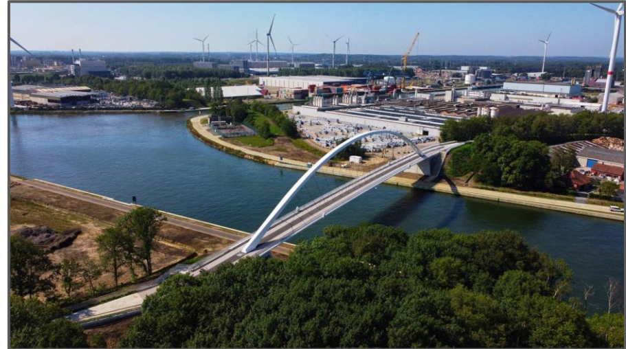
Figure 11 - Bicycle bridge at Tessenderlo, Belgium Anker. (n.d.). Bicycle Bridge Tessenderlo, Belgium. Anker.
