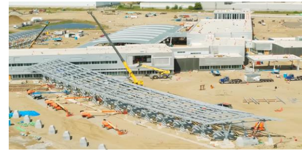
Figure 19. Prefabricated Girder panels
