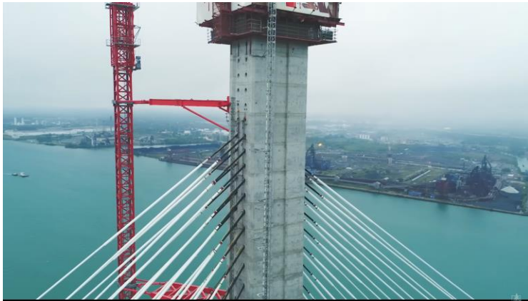
Figure 17. Anchors at pylon for cables
