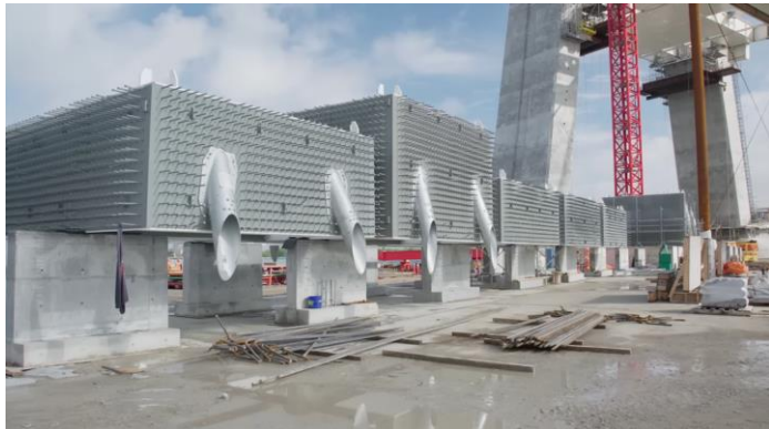
Figure 15. Steel boxes in upper pylon
