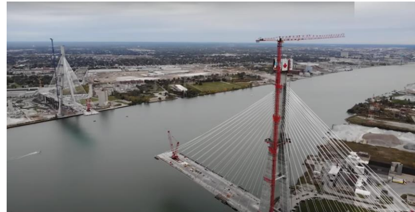
Figure 14. Construction of Gordie Howe Bridge
