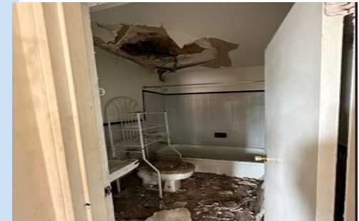
Collapsed ceiling in a bathroom of Arverne Unit
