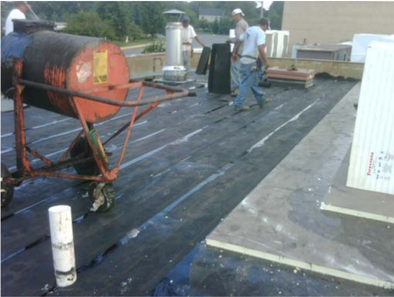
Coal Tar Roof
