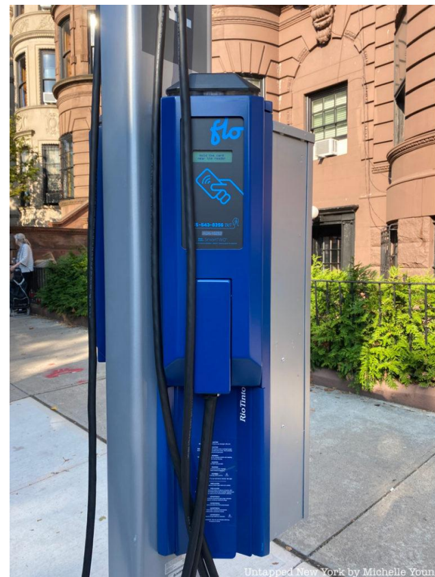
Image of a level 2 charger in NYC Source: Untapped New York, Michelle Young, 2021
