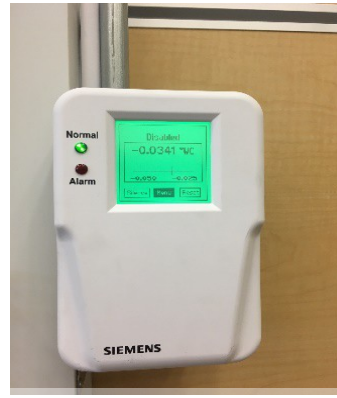
Diff. Pressure Monitor, tied to building BMS
